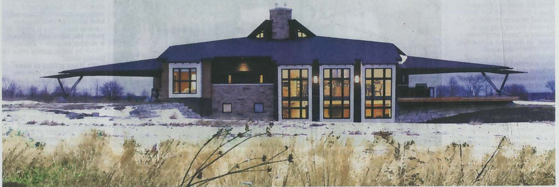
Two wings resembling triangular carports extend from two corners of the house. The first shapes how the wind travels around the house; the second influences how it leaves: 'It's sort of like the [Toyota] Prius ... it sort of has that slope,' Mark Driedger says. Windows are precisely angled to maximize seasonal heat loss or retention. MARK J. DRIEDGER
